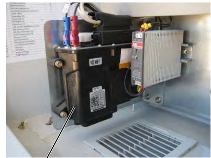
LiTU – Box (Liebherr T elematic U nit)
